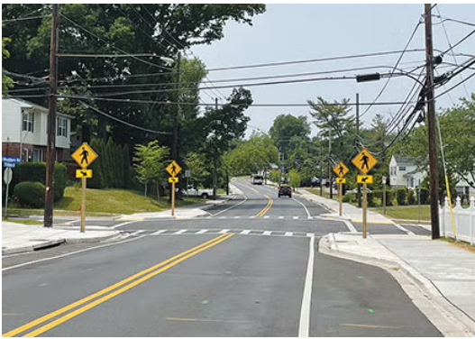
Figure 44. Concrete Curb Extensions
