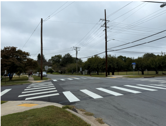
Figure 12. High-visibility crosswalks at Congressional Lane / Lorraine Drive and Rollins Avenue
