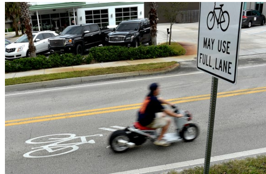
Figure 42. Shared Lane Markings and Signage
