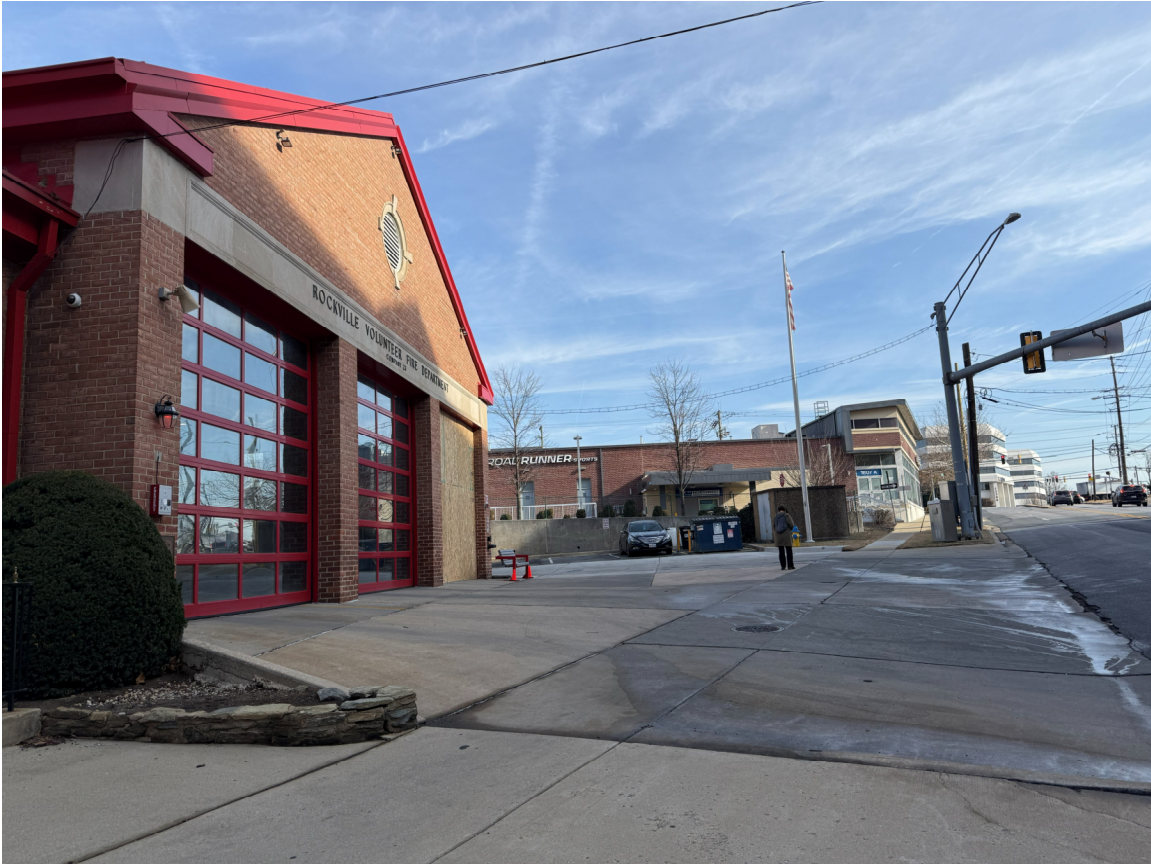
Figure 37. Fire Station on Rollins Avenue near Rockville Pike (MD 355)
