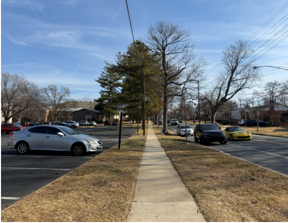
Figure 20. Four feet wide sidewalk in the residential segment
