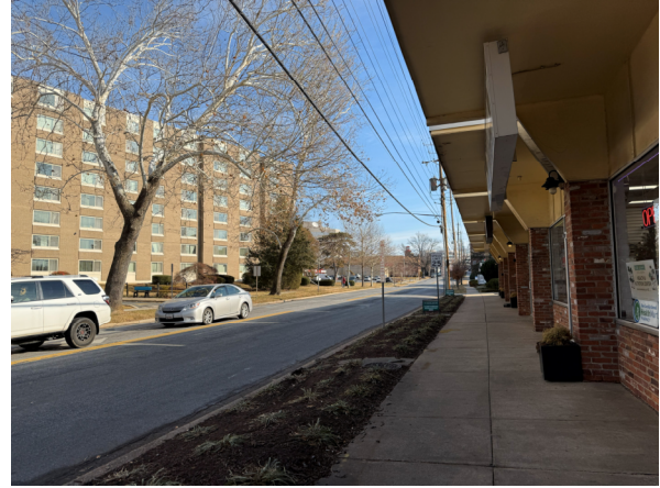
Figure 21. Sidewalk widens to eight feet on the south side of Rollins Avenue, east of East Jefferson Street
