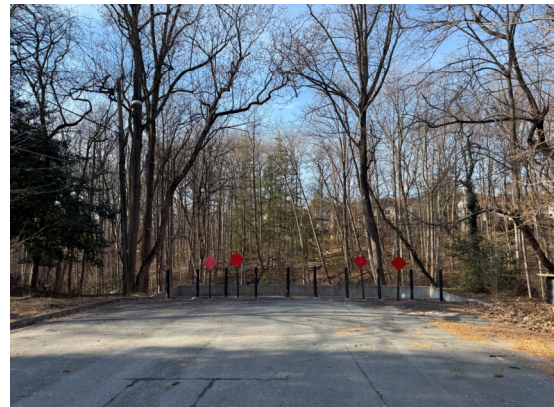
Figure 15. Roadway end at Old Farm Creek
