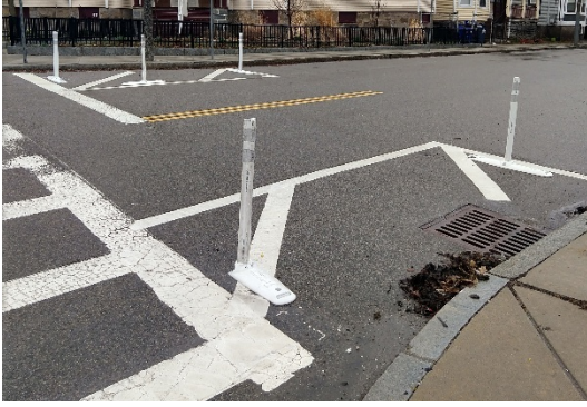
Figure 43. Painted Curb Extensions and Flex Posts
